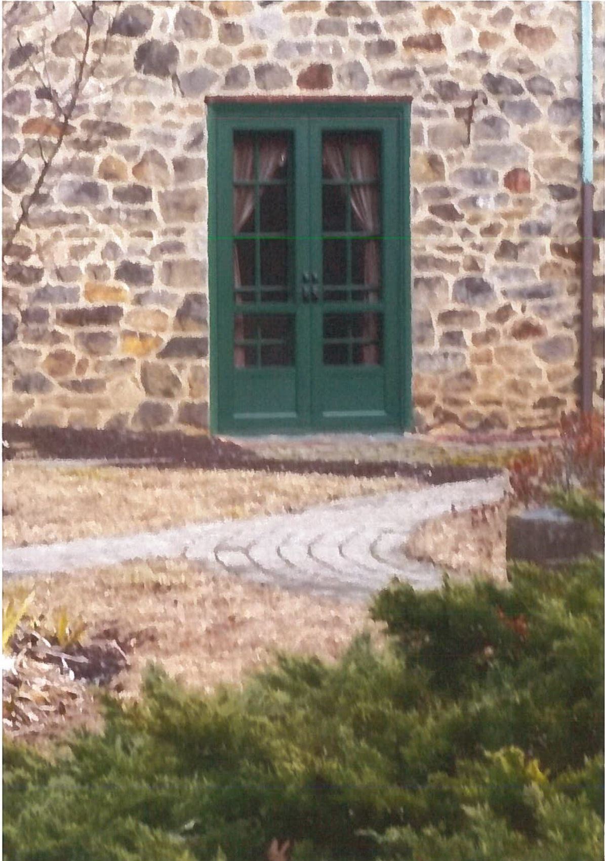
Residential Secondary Door 46 East Market Street Bethlehem, PA
